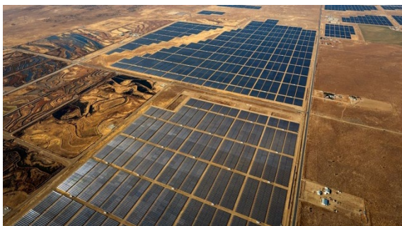
Image 3: Solar panels collect the sun's rays and turn them into electricity for us to use everyday.
