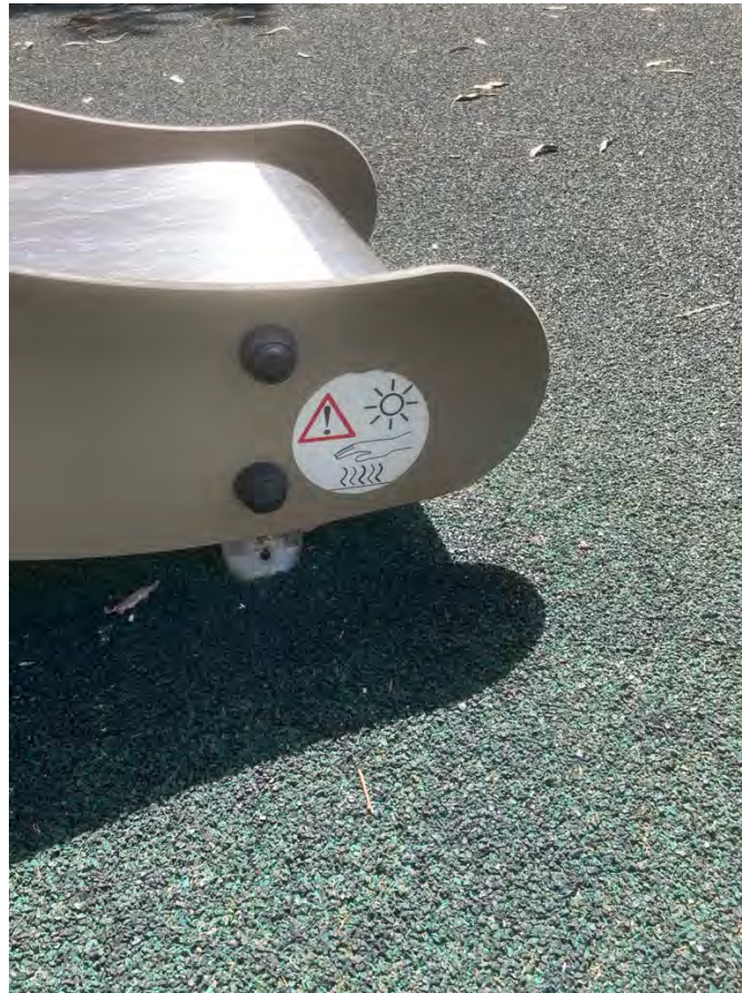
Figure 7 Only one of the local slides had a warning sticker, it was one of the metal slides
